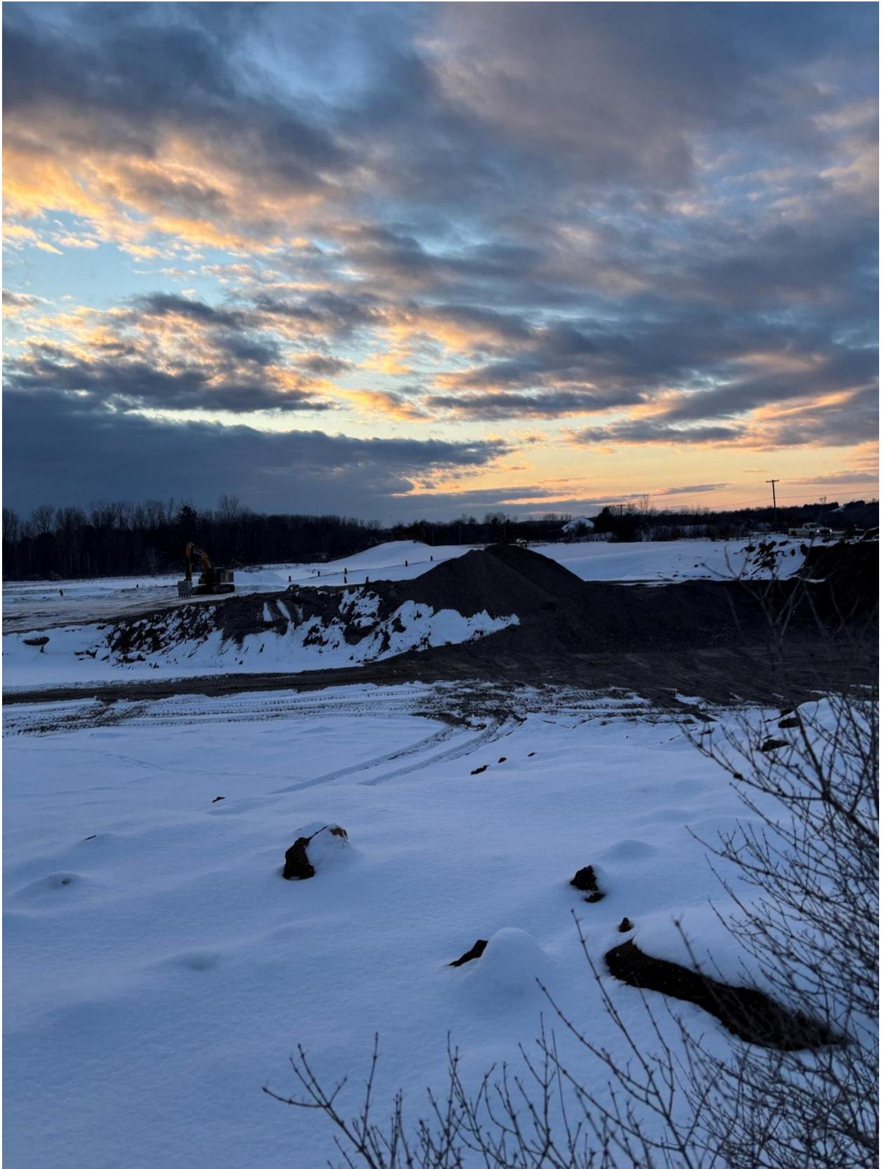
This picture Taken January 27 th 2025 shows the depth of the excavation of the Rural Residential Lots on Little Lake Rd and Trent Vally Road and the stockpiled fill yet to be withdrawn.
