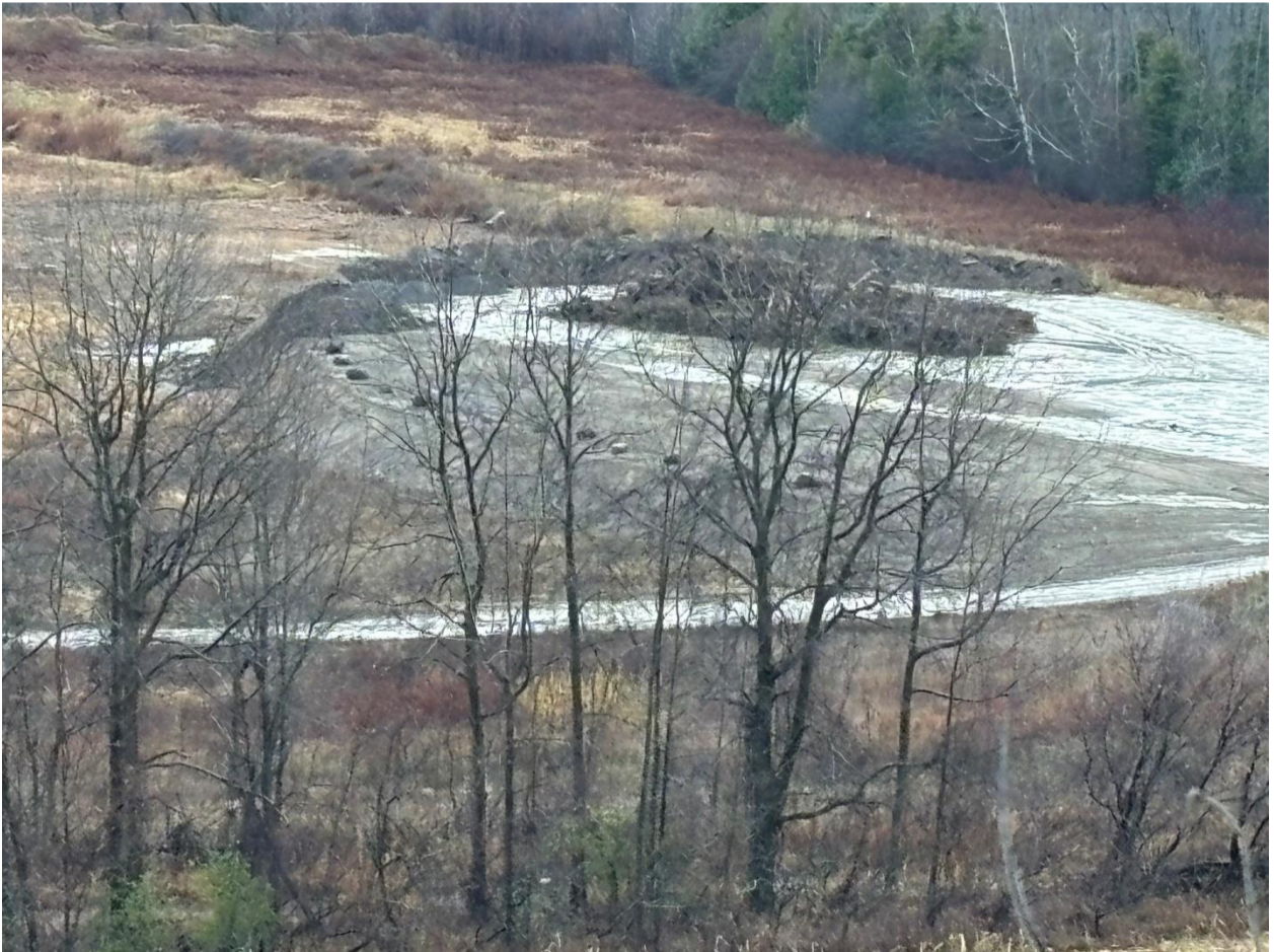
This picture shows the extensive build up of fill, rubble, trees and brush in the area where excavation of gravel went below the water table at the most southerly end of the Pit. The built up area is assumed to be the foundational area for the plant. This picture was taken November 22, 2024 after a light Rain.
