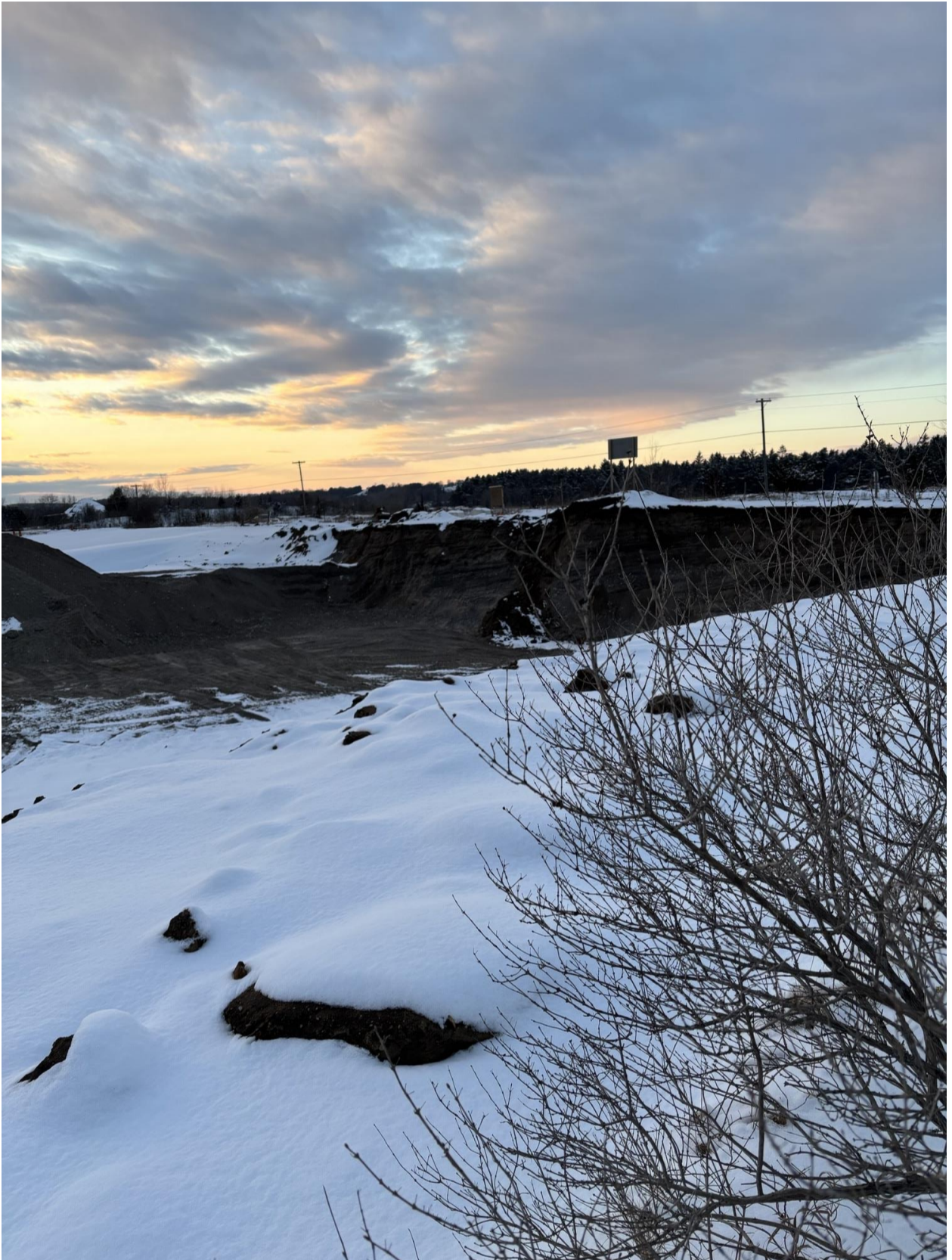
This picture Taken January 27 th 2025 shows the depth of the excavation of the Rural Residential Lots on Little Lake Rd and Trent Vally Road. The depth of the excavation is approximately 40 ft. The sign seen at the top of the picture is at road level.
