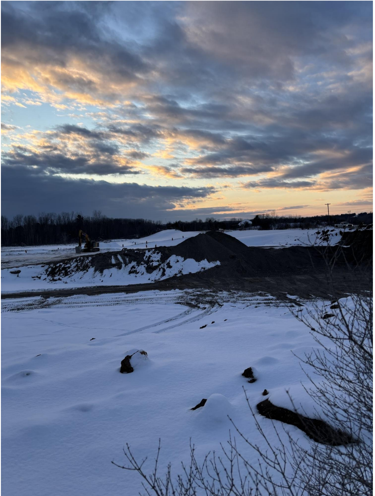
This picture Taken January 27 th 2025 shows the depth of the excavation of the Rural Residential Lots on Little Lake Rd and Trent Vally Road and the stockpiled fill yet to be withdrawn.
